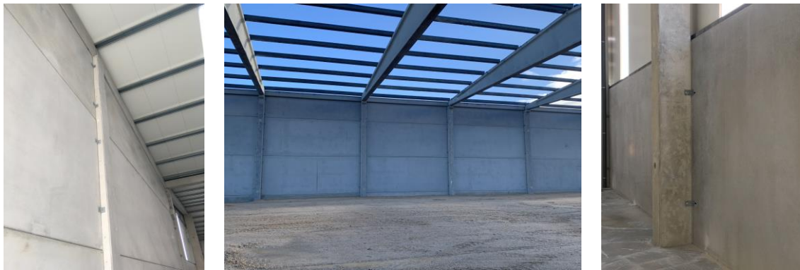
Figure 1 - Typical Portuguese industrial building with horizontal cladding panels.
