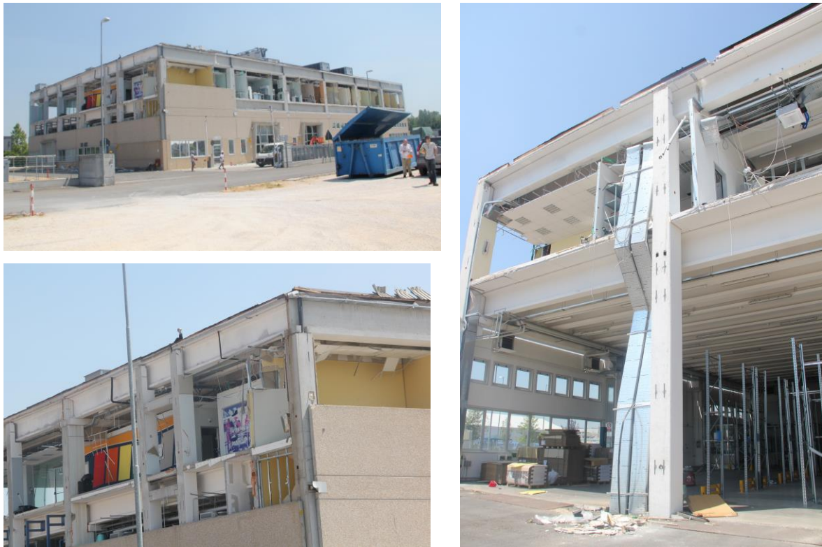
Figure 3 – Precast cladding failures.
