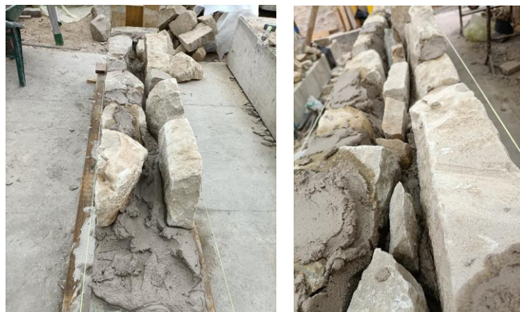
Figure 2. Construction of the double-leaf stone masonry walls.
